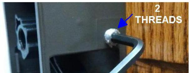
4. Make a note of the orientation of the cam. The opening of the cam should be directed toward the landing door. It is important that you install the new metal cam in the correct orientation.
