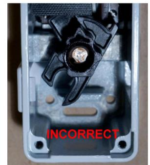
5. Remove the plastic cam by rotating it toward the elevator car. When the arrow on the cam is pointing up, you will be able to pull the cam off the shaft.
